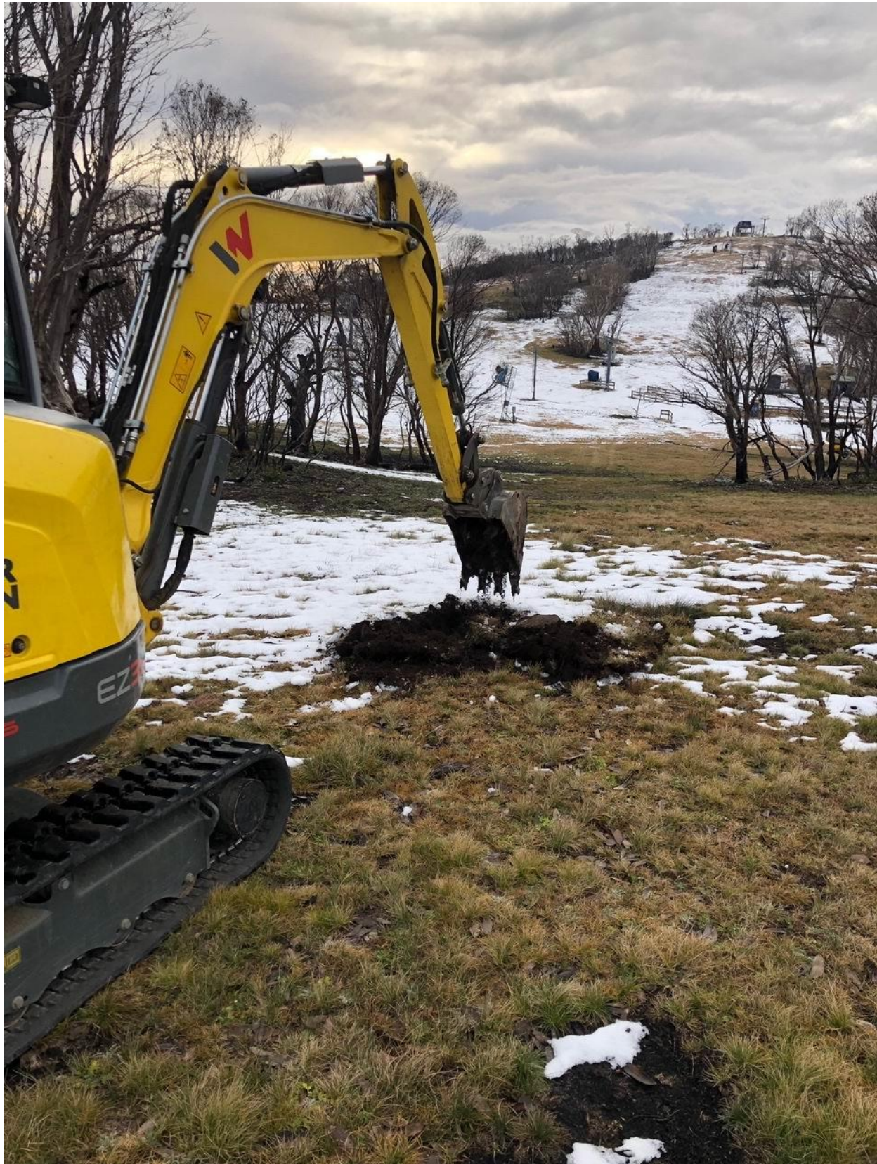
Photo 7 – 10/7/2020 – View of test pit 3T being excavated.
